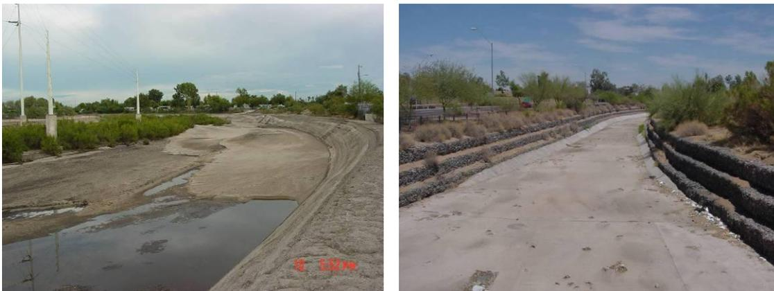
**Figure 3. Stream channelization and bank stabilization structures along two rivers in Arizona (photos courtesy of G. Zaines (left) and D. Green (right)).**
